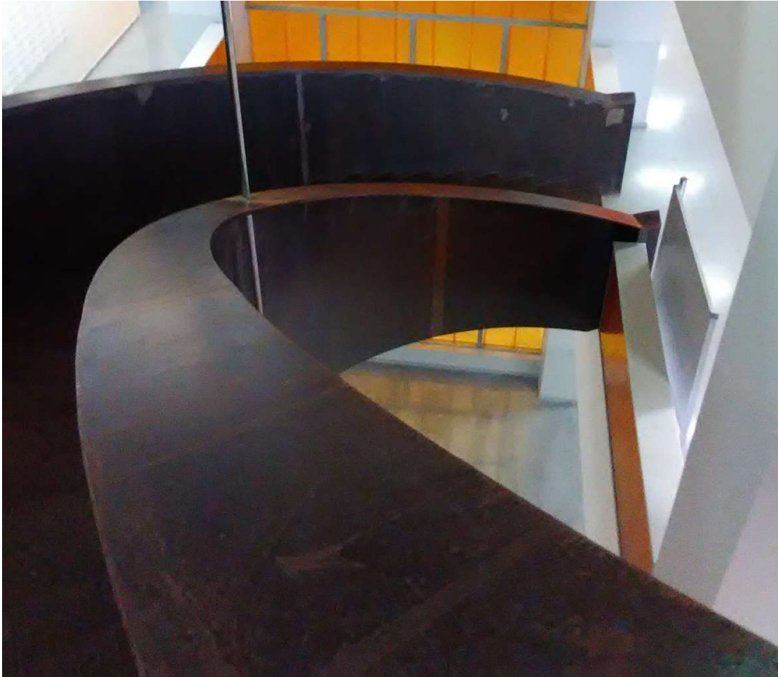
Figure 00. Main stairs of Engineering School of Bilbao II. Picture made by the authors, 2018.
