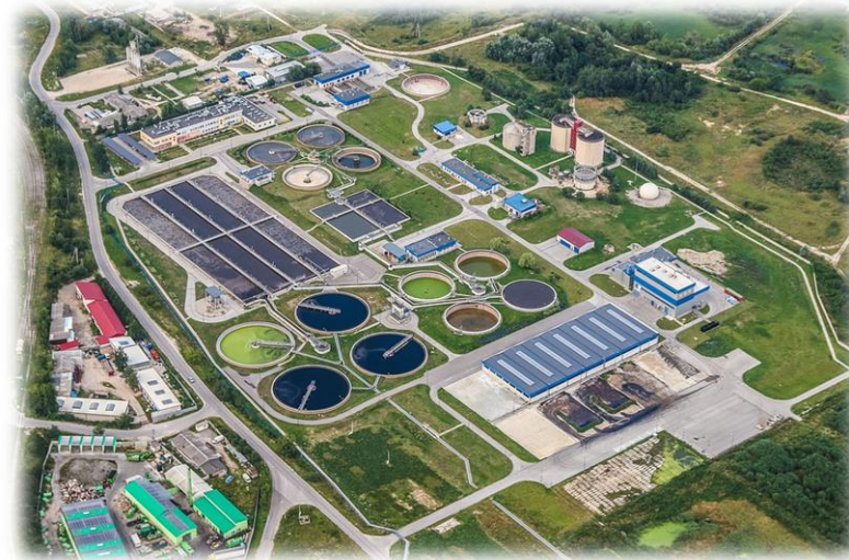
Wastewater treatment plant by Michal Jarmoluk from Pixabay licensed under CC0
