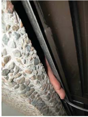
Figure 13: Dismantlement of interior finishes at window head reveals direct air leakage path.
