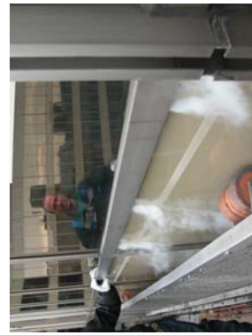
Figure 13: Dismantlement of interior finishes at window head reveals direct air leakage path.
