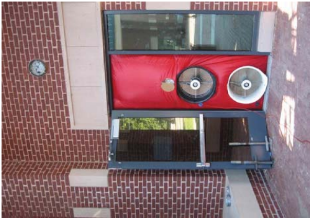
Photo 2: Test setup for blower door test with calibrated fans.
