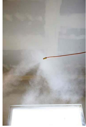
Figure 6: Photo of sealant atomization
