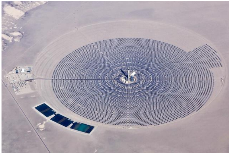
Fig. 22. Crescent Dunes Solar Energy Project, Tonopah, Nevada. [Iturri]
