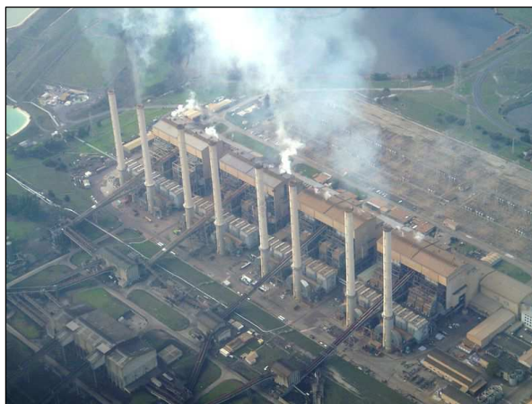
“Fugitive emissions at a Power Station” by Mriya licensed under CC BY-SA 3.0
